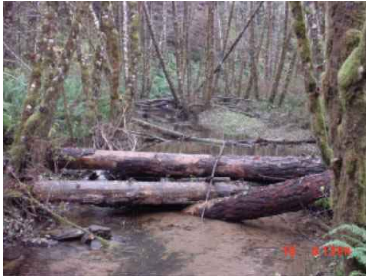
Big Creek after log and boulder structures have been placed.
