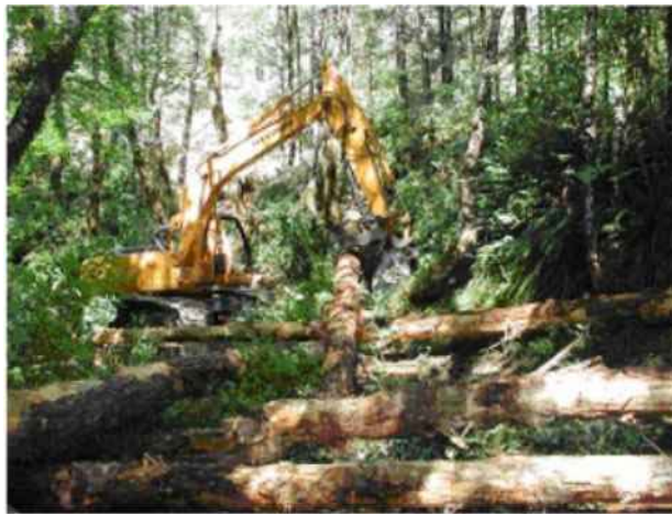
Figure 1 Constructed log jam on Big Creek
